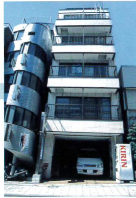
▲3号館 Annex Building
