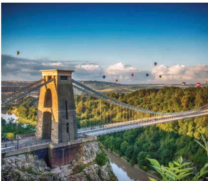
Clifton Suspension Bridge, Bristol
