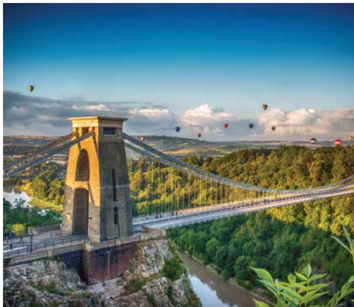
Clifton Suspension Bridge, Bristol
