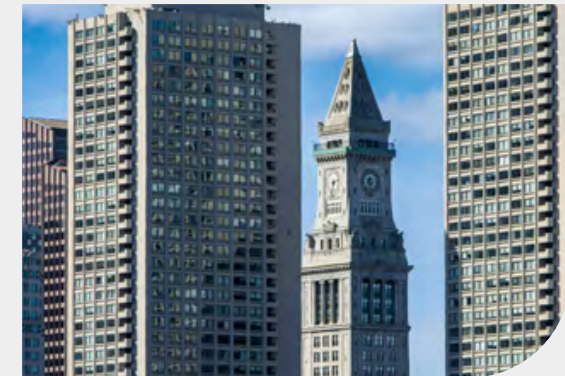
Boston financial district, McKinley Square, Custom House Tower
