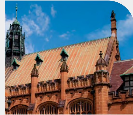
The University of Sydney, building detail
